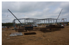
Newton Aycliffe, UK production site: Under construction
