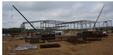
Newton Aycliffe, UK production site: Under construction
